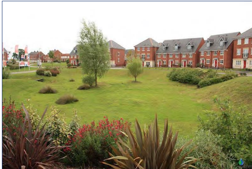
Figure 3.15 - Example Detention Basin
